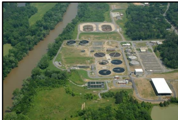
Figure 2. Rome Water Reclamation Facility
